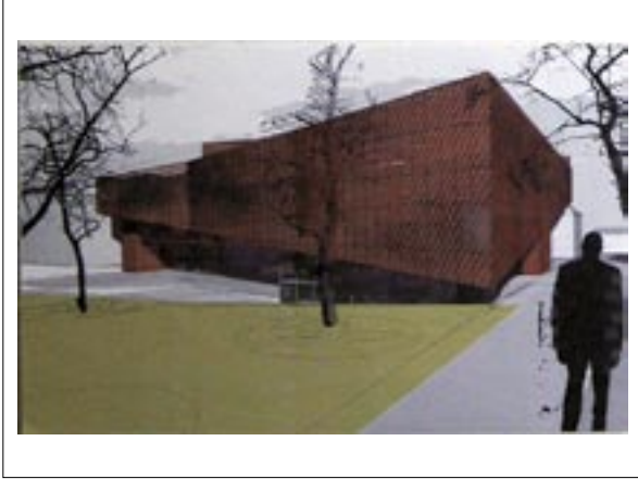
Original design - front facade The volume of the auditoriums does only touch ground with the necessary circulation elements. The transparent facade is hanging above ground.
